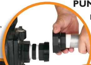
2. Connect the new pipe to pump by winding the Common Centre Nut onto the matching male thread
