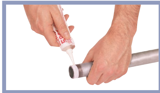
1 (b) thread paste sealant. The right sealant for threaded joints is non-hardening, compatible with plastic and doesn't add slipperiness to encourage over-torquing.
