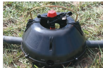
Flush the irrigation line prior to fitting the pipeline end cap to remove any drilling debris left in the pipe.
