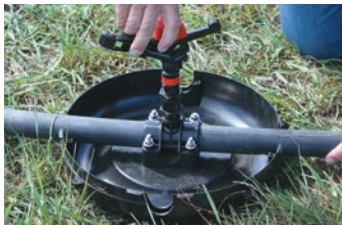
Screw sprinkler into Hansen Socket on riser.
