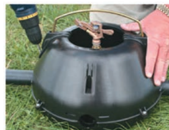
Screw wire clip holders into the holes provided.
