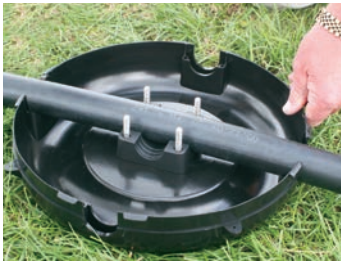
Lay pipe over Skid Base and secure in position with Cross Tee Anchor.
