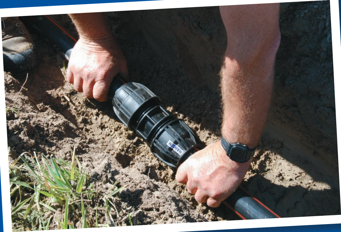
Hansen Medium Density Coupling (HMDC) in use
