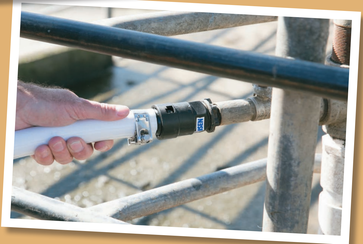
Hansen Quick Release Coupling (HQC) in use
