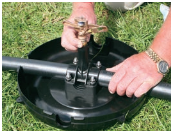
Screw sprinkler into sprinkler riser.
