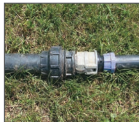
Step 6. Disconnect the Drag Hose from 90mm Adaptor Set and drag to new paddock.
