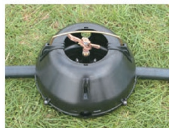
Flush the irrigation line prior to fitting the pipeline end cap to remove any drilling debris left in the pipe.
