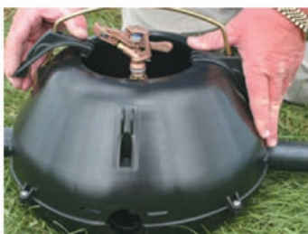
Fix wire clip into opposing holes on body sides. Ensure the wire runs parallel with the pipe as shown in the image.
