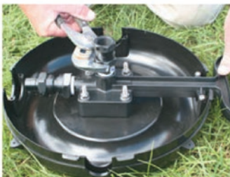
Insert the Hansen Hex Nipple into the Pod Skid Base. Then screw on the Hansen 20mm Female Socket.
