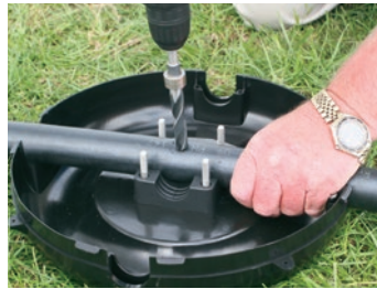
Drill 15mm (9/16") hole at required spacing for the sprinkler type being used and remove all drilling swarf. Ensure the hole is drilled perpendicular to the Pod Base.
