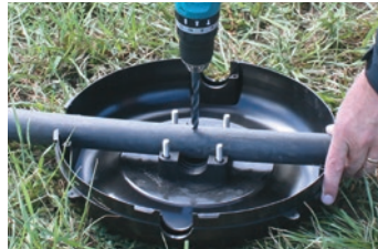
Drill 15mm (9/16") hole at required spacing for the sprinkler type being used and remove all drilling swarf. Ensure the hole is drilled perpendicular to the Pod Base. Caution: Do not drill through both edges of the pipe.
